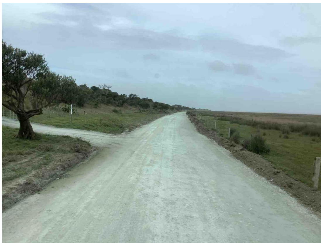
Overlays continuing on North Road.
