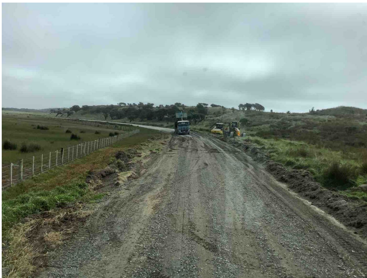
North road strengthening.
