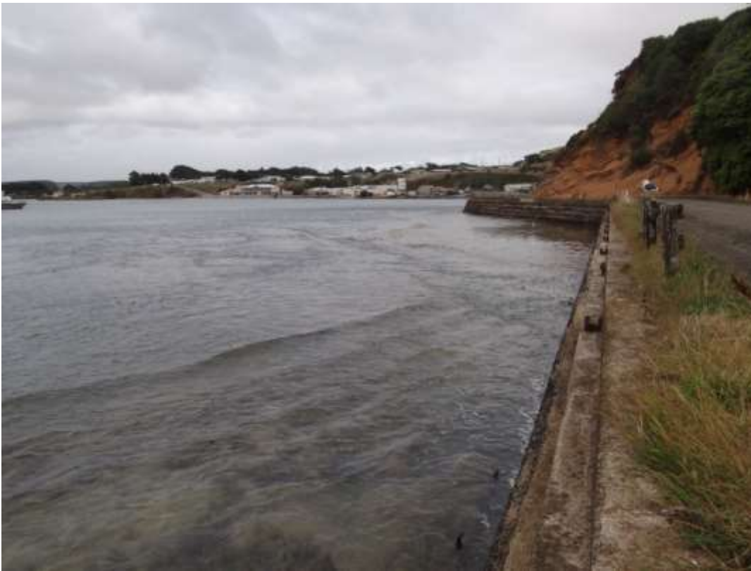
Figure 2-19 Road seawall reflecting oblique incoming waves towards the beach
