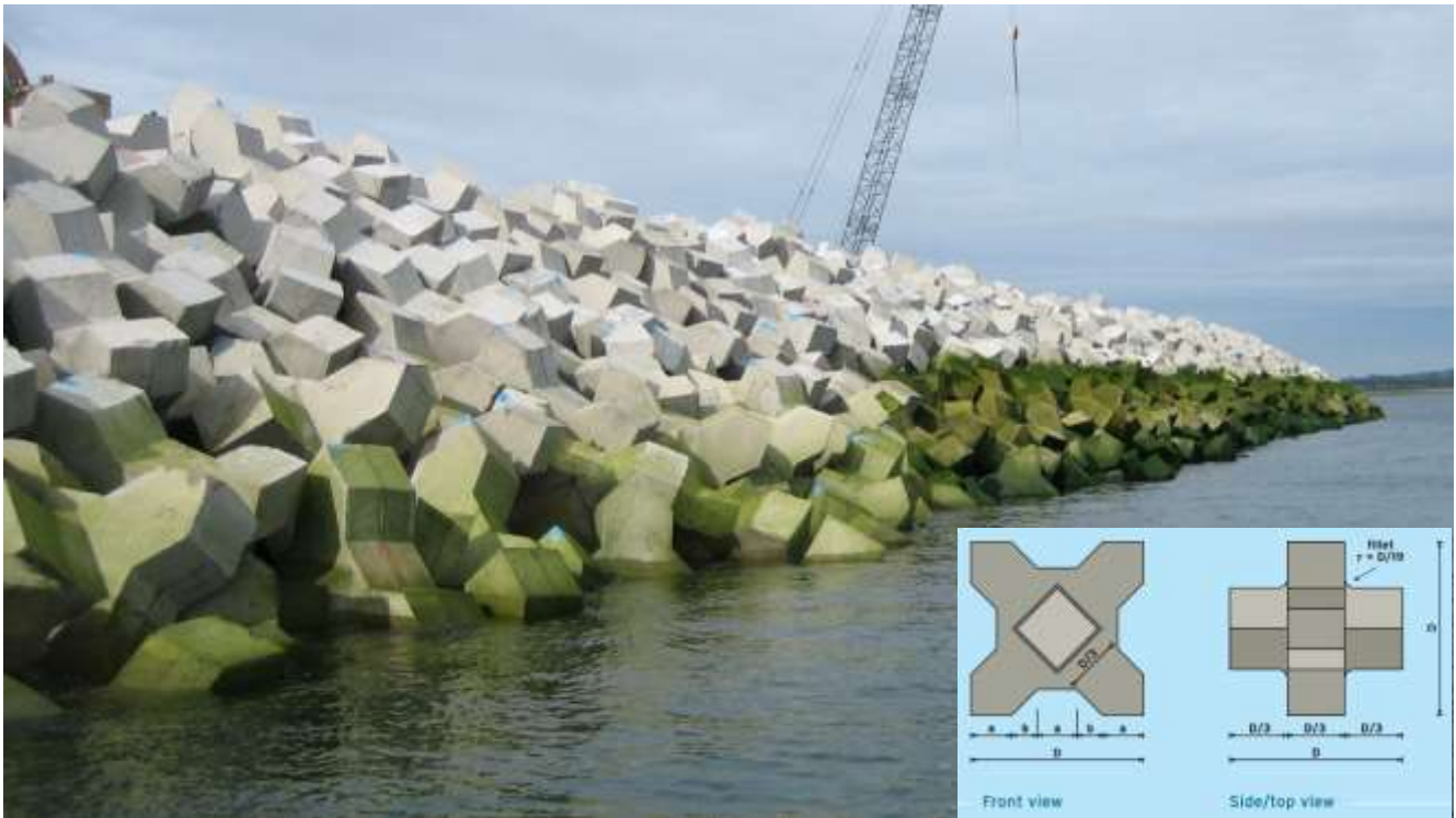
Figure 3-2 Example of breakwater constructed using Xbloc armour units (source: DMC, 2013)
