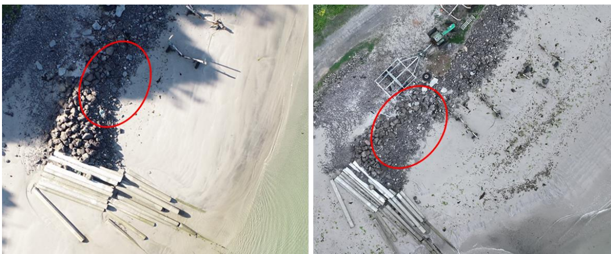
Figure 3.3: UAV images (2022 left and 2024 right) at point 1 showing increased displacement of access ramp rock armour
