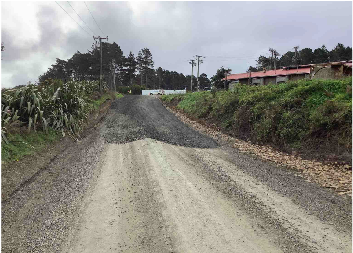
Corner Widening And Anti Scour Works On WW-O Road
