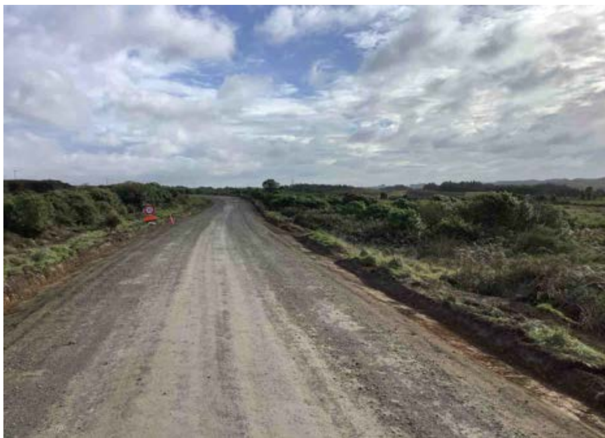
Watertabling WW-O Road
