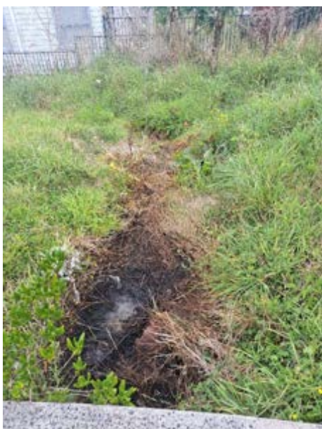
Fig. 65: Discharge point to swale that leads to creek, showing staining. This swale leads to a coastal marine area (CMA).
