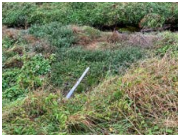
Fig. 22: Outlet pipe discharging to creek.
