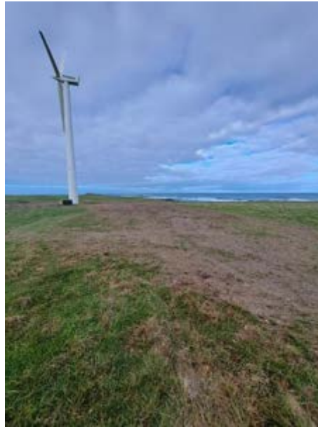
Fig. 94: Reprofiled ground following installation.
