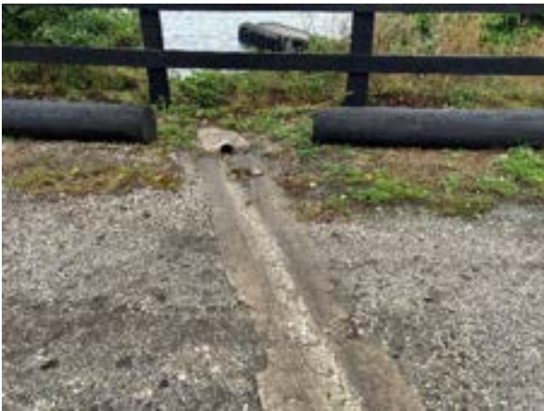
Fig. 18: Stormwater outlet to coastal marine environment.
