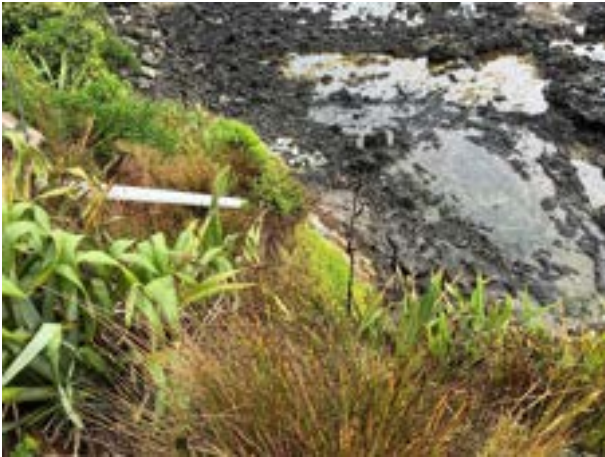
Fig. 16: Outlet pipe discharging to coastal marine environment.
