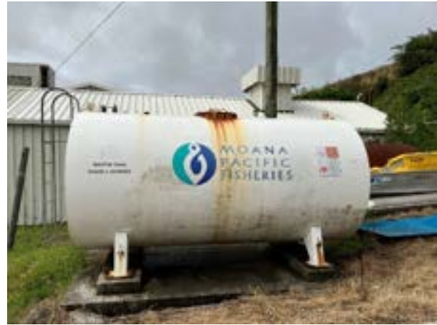
Fig. 8: Double skinned, 10,000L diesel tank.
