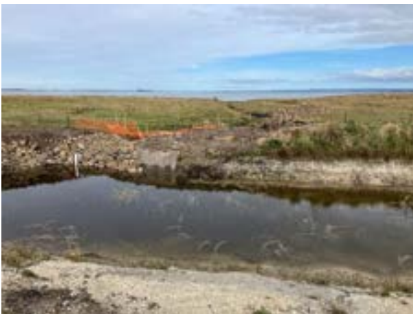
Fig. 28: Stormwater retention pond.
