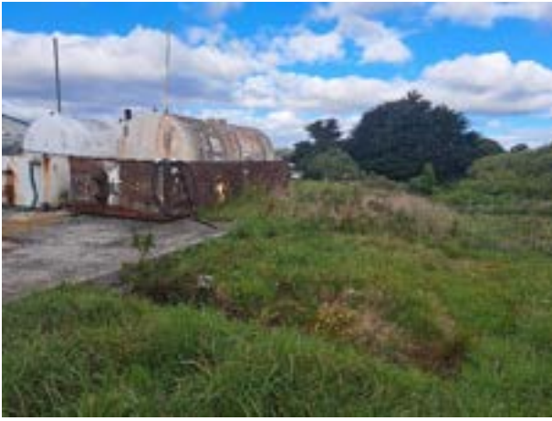
Fig. 67: Impacted swale that leads to creek, which in turn discharges to CMA.
