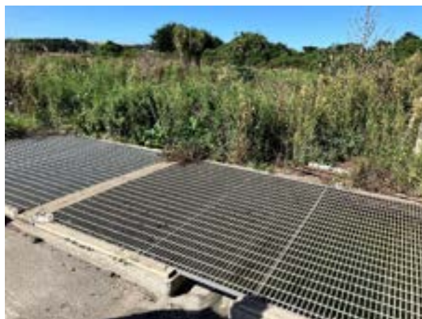
Fig. 59: Truck wash storage tank.
