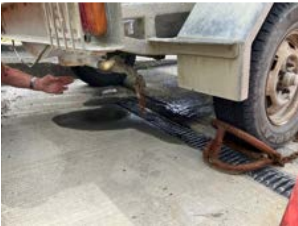
Fig. 26: Oil spill from mobile fuel tank into strip drain.
