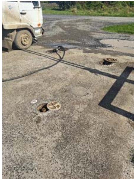
Fig 70: Two tanks being refilled at time of visit.
