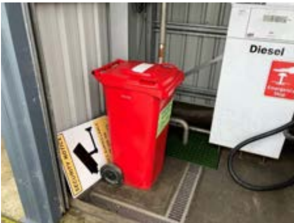
Fig. 77: Spill kit for diesel bowser.
