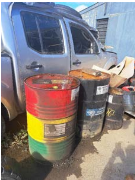
Fig. 30: Waste oil drums stored on ground outside workshop.
