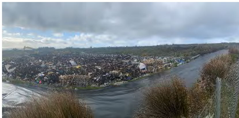
(Liner at the Northern wall before being covered with Geotech and soil )
