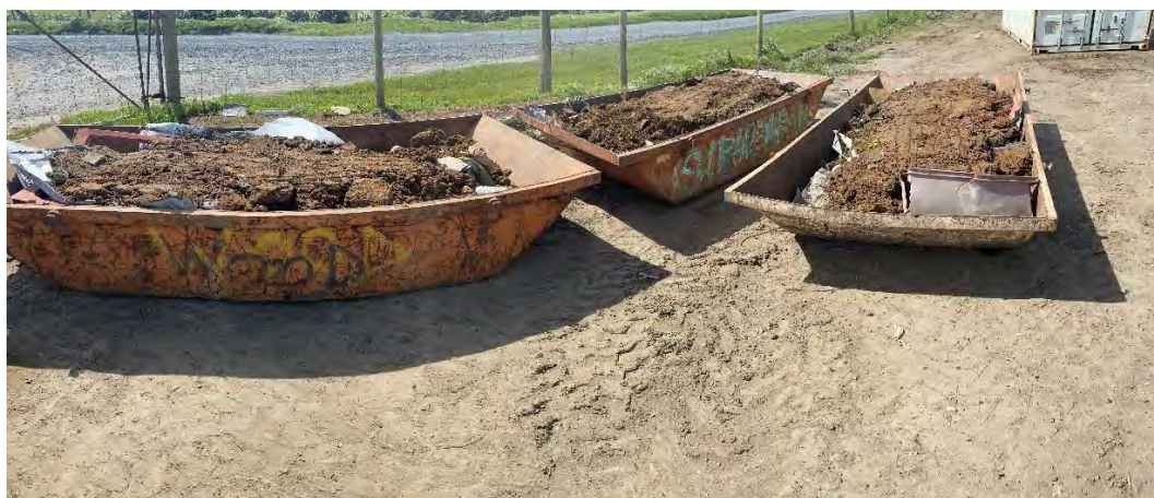
( Skip bins filled with waste scrap metal and soil cover, ready for transporting )
