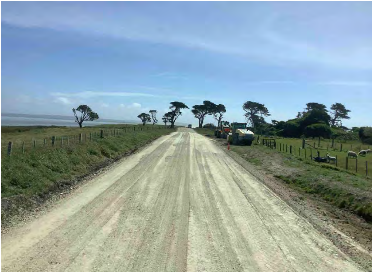
RP 35500 – 36400 North Road Strengthening Works
