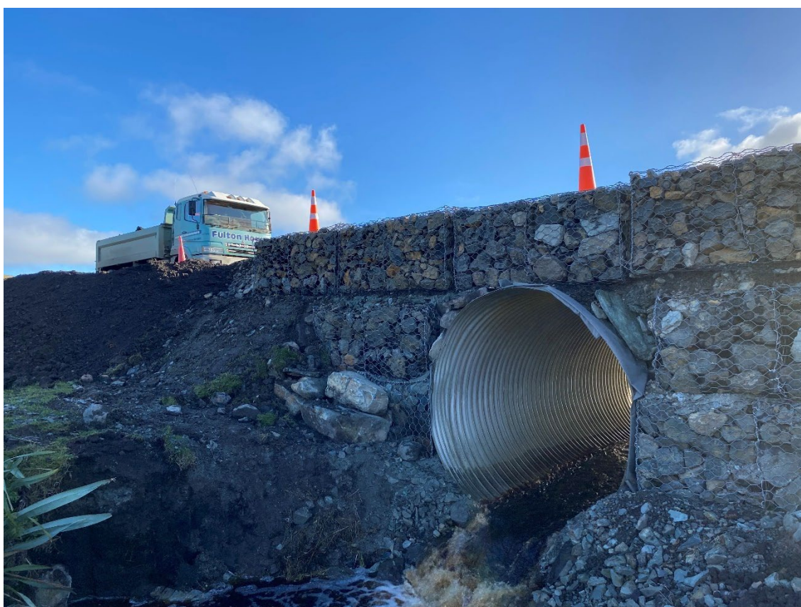
Gabion baskets completed at Waikawa Culvert
