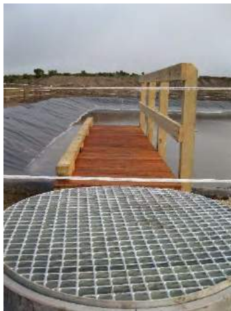
Figure B3-3: Leachate pond outlet structure.
