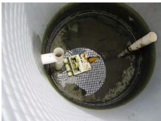
Figure B3-5: Overflow flout to discharge leachate to the pilot plant.
