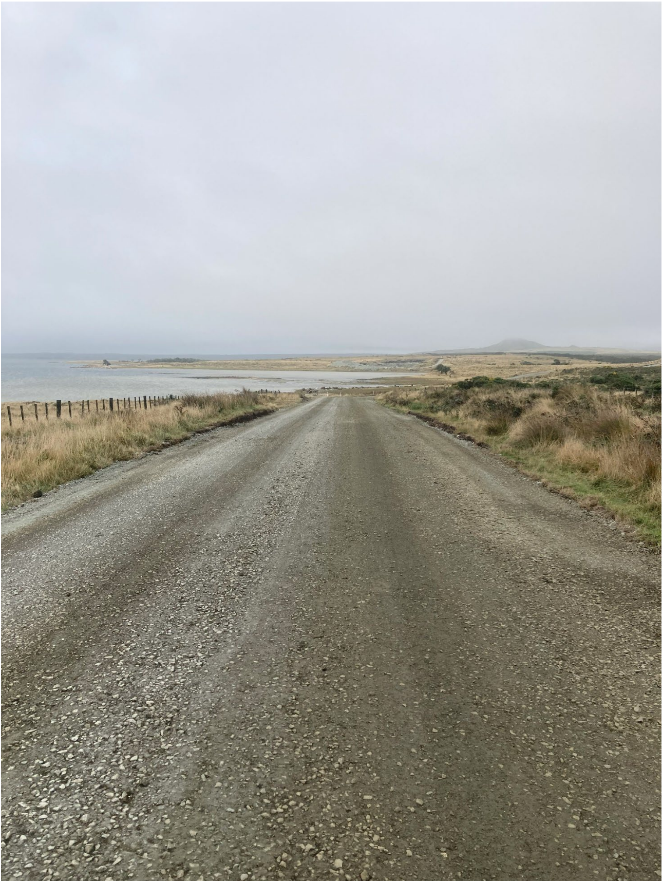
North Road Strengthening Works
