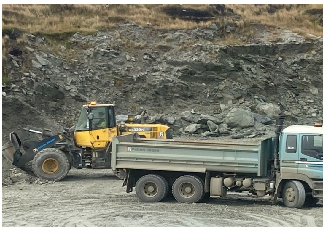
Loading Truck In Waitaha Schist Quarry
