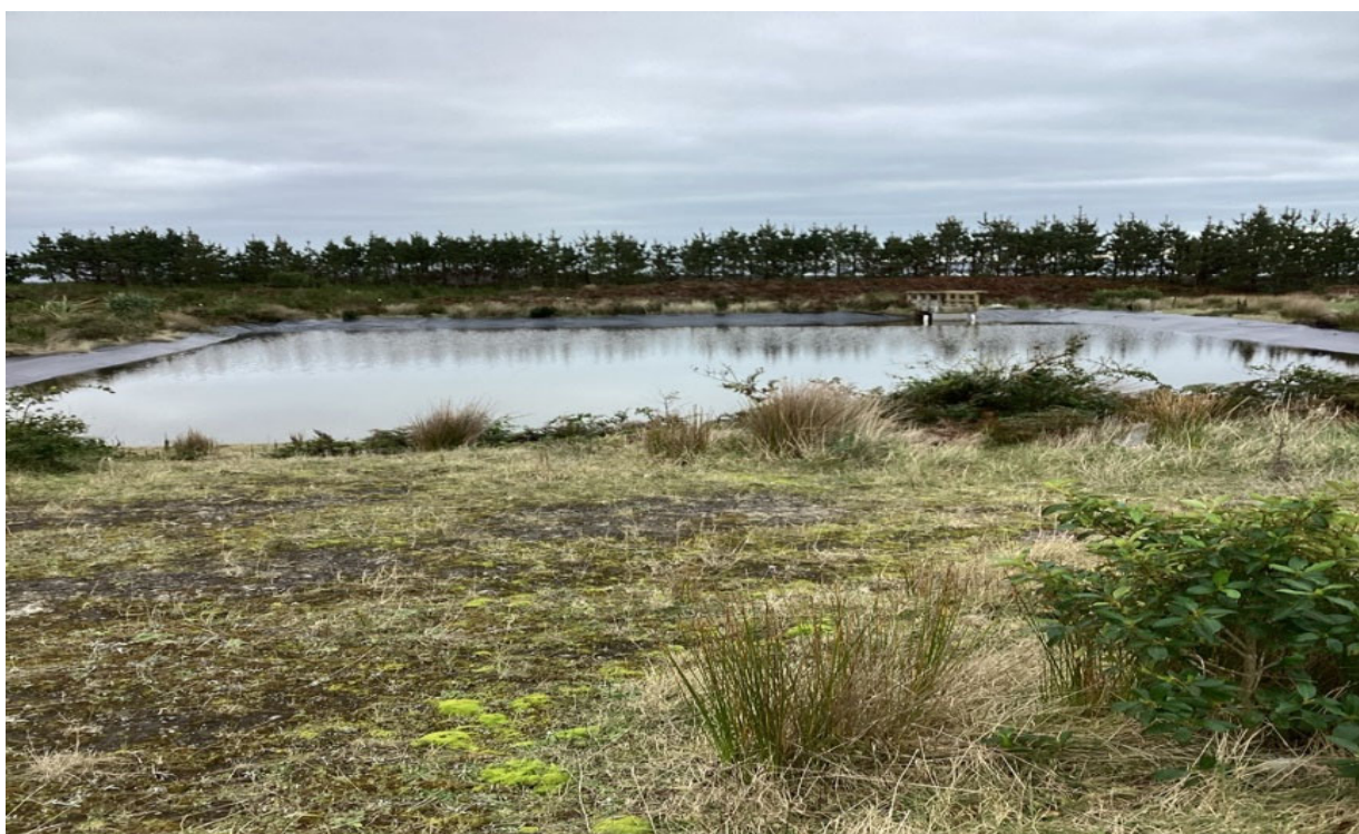
Owenga Leachate Pond
