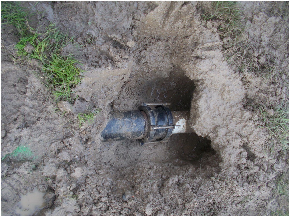
One of the many joins in the sewer line near the solids tank
