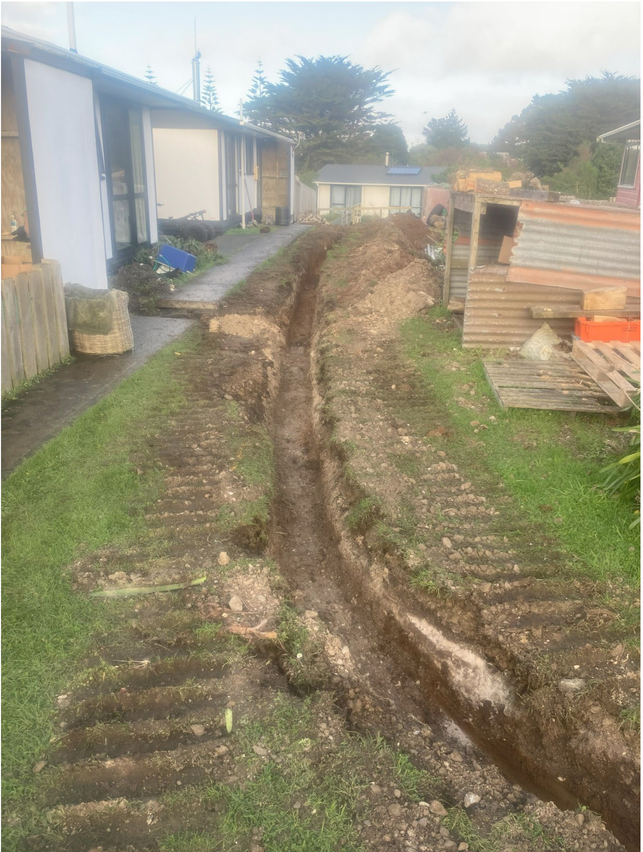
Trenching at The Council Flats.
