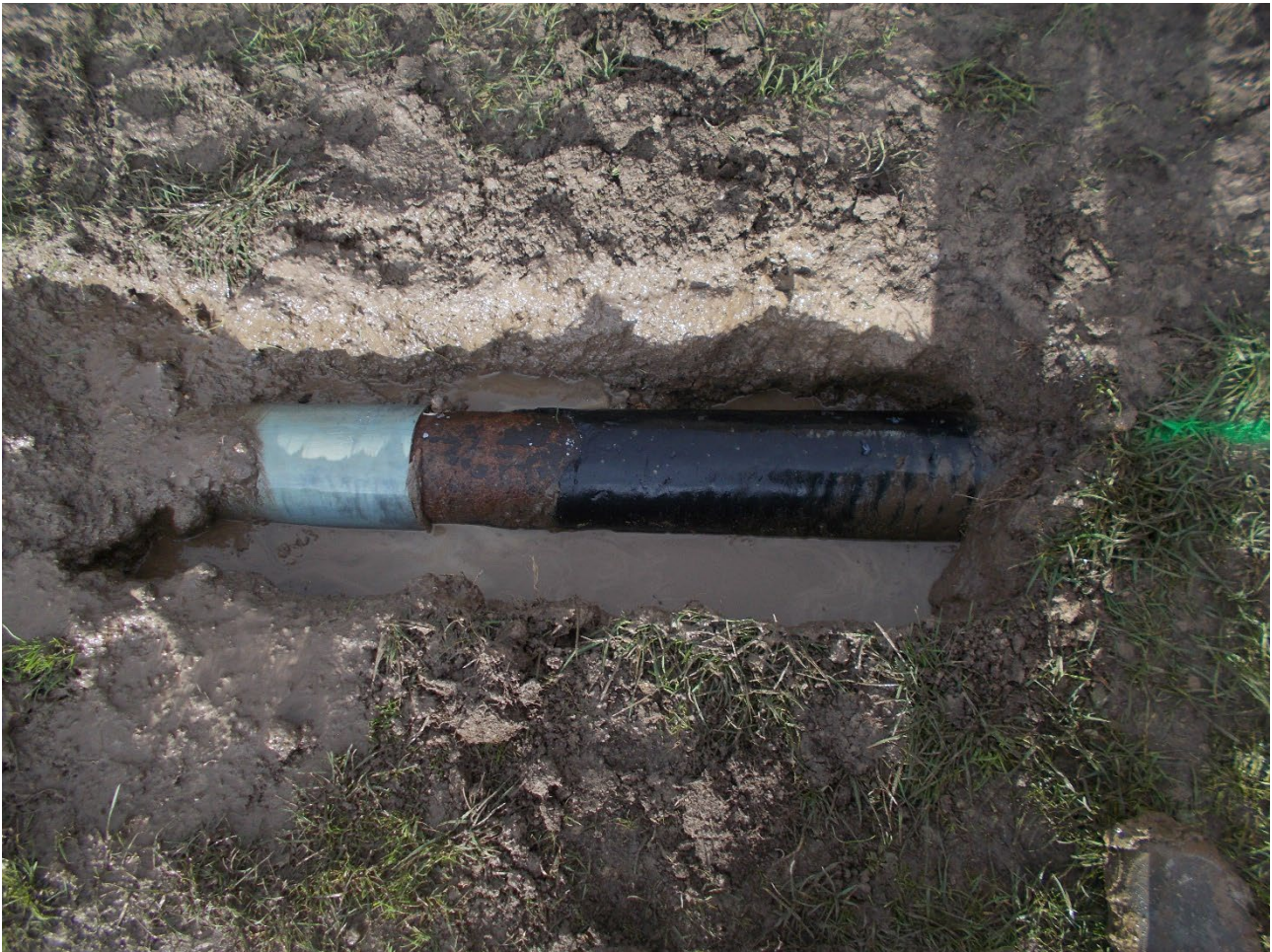
Another join by the solids tank in Waitangi.
