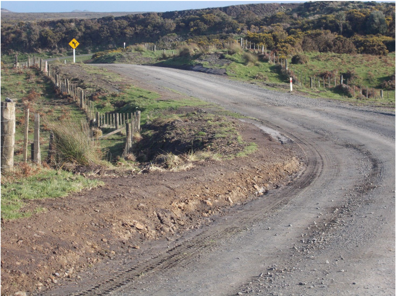
Area of north Road ready for strengthening.
