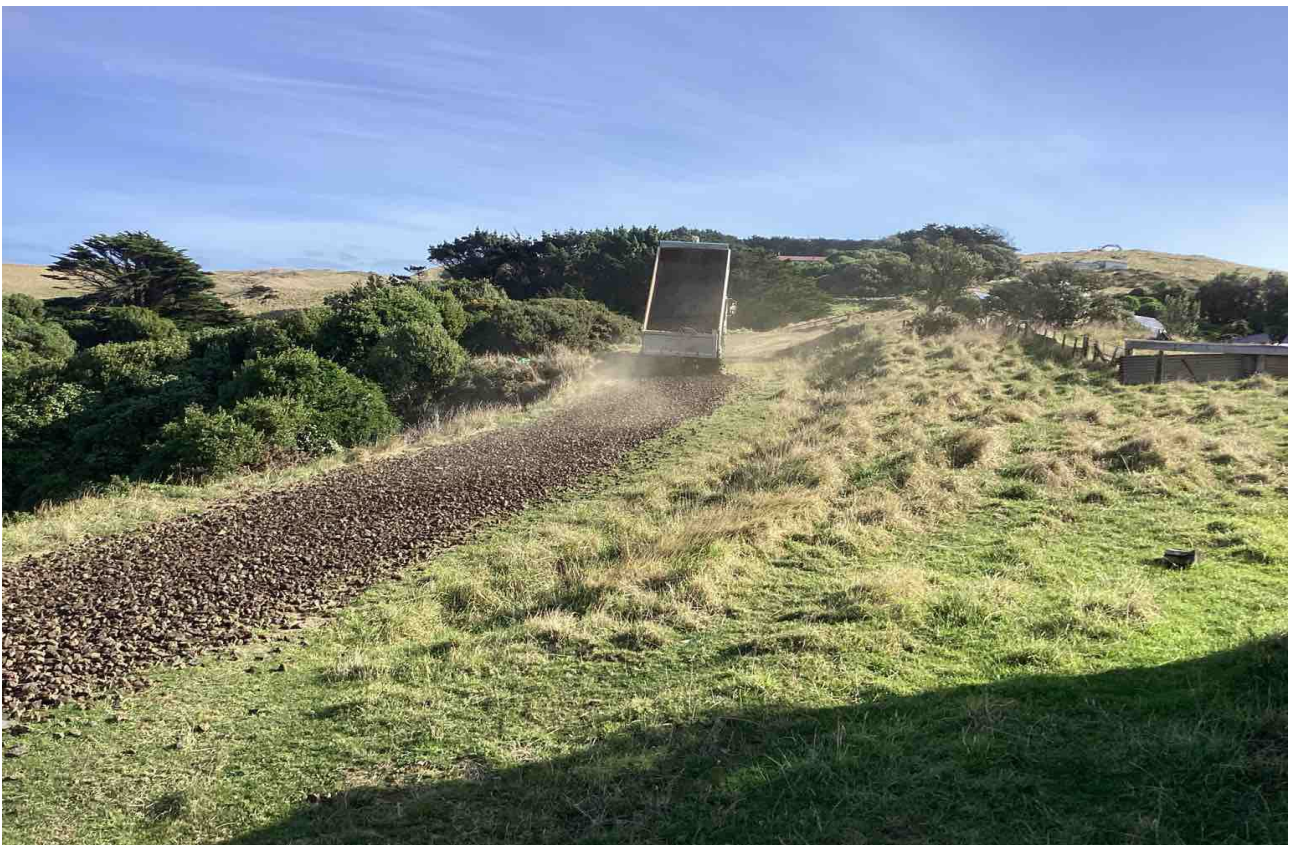
Maintenance Metalling Unerway On Pitt
