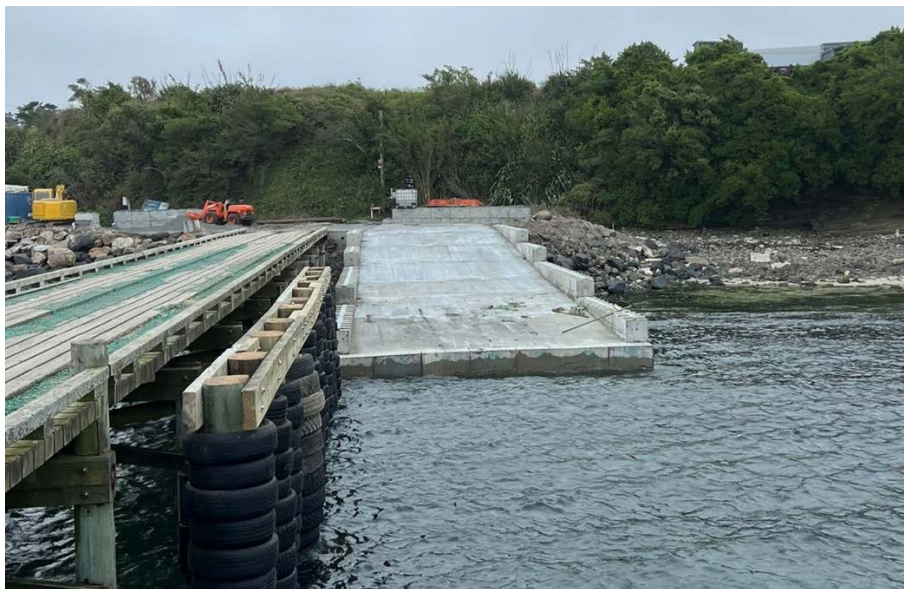
Figure 1 New barge loading facility and fender system
