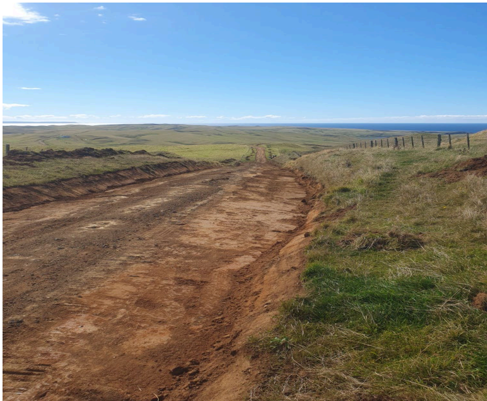
Watertabling On Pitt Island
