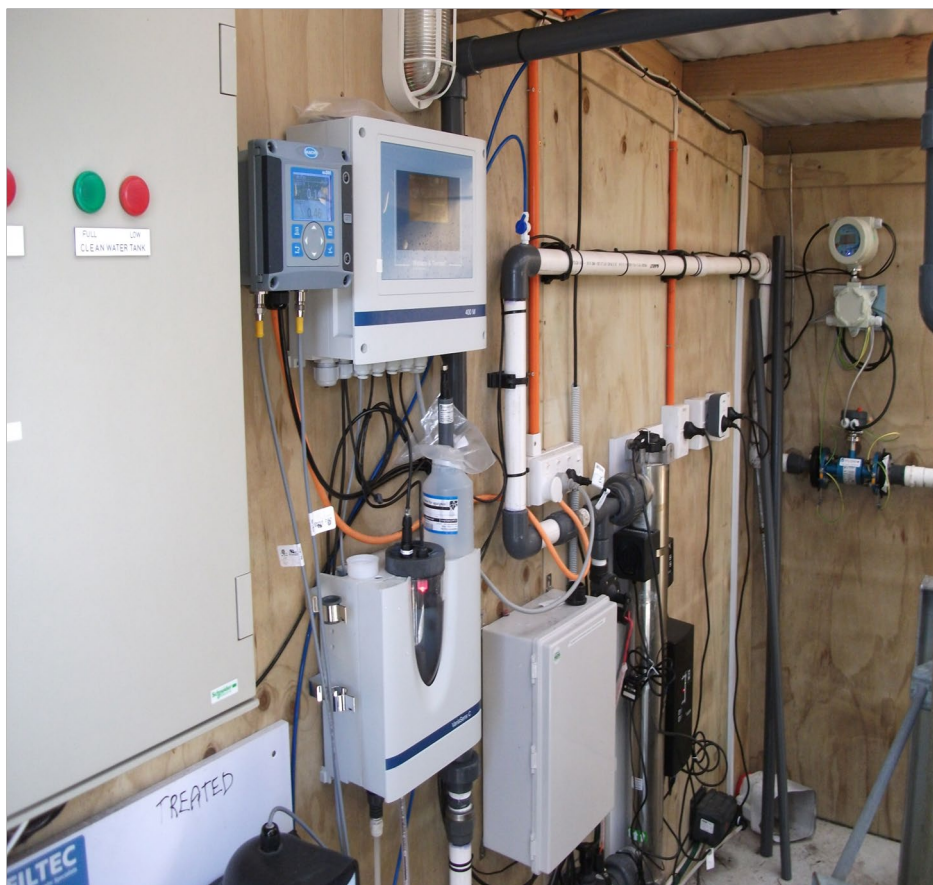
Kaingaroa Water Plant
