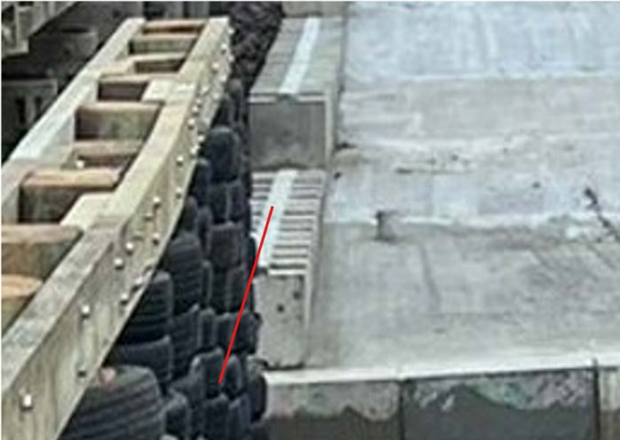
Figure 3 Interbloc to barge door ramp clash location
