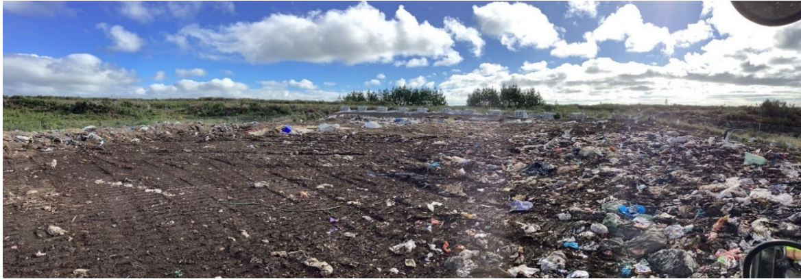
Photo of track rolled wastes and soil cover spread over pad to hold waste down.
