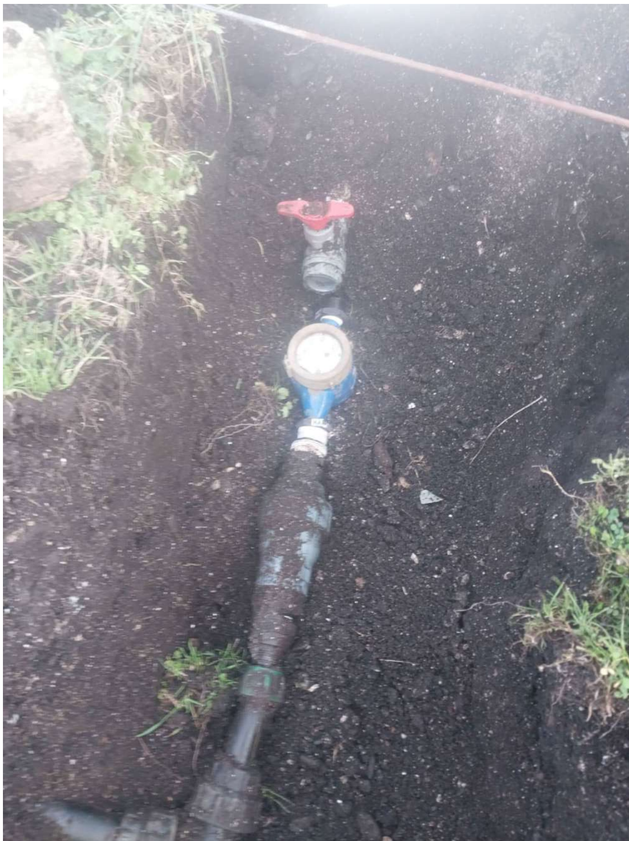
Installing new meters at Kaingaroa farm tanks.
