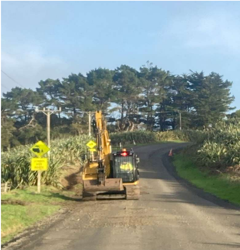
Clearing Watertables WW-O Road
