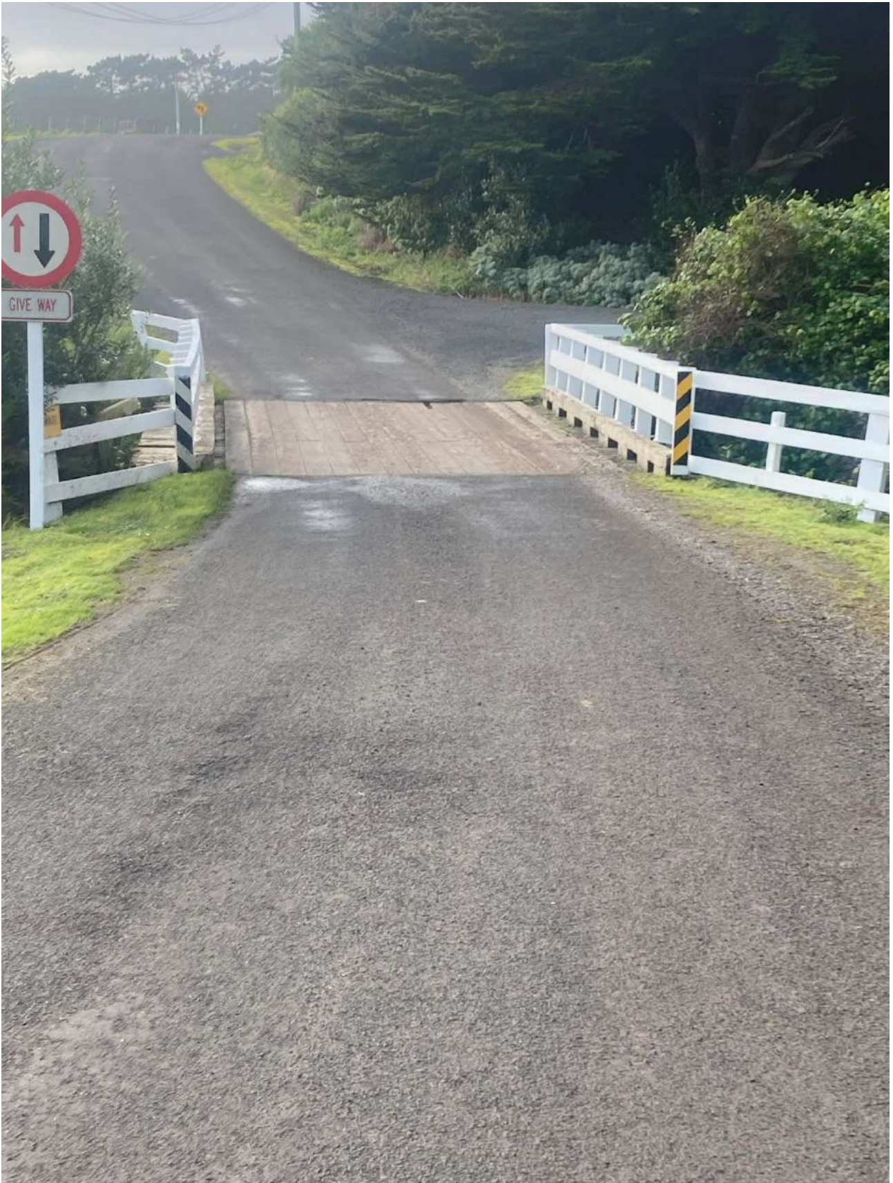
Fresh coat of paint on all the bridges.
