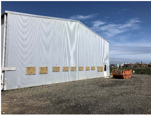
Figure B2-1: North-western side of the MPB.
