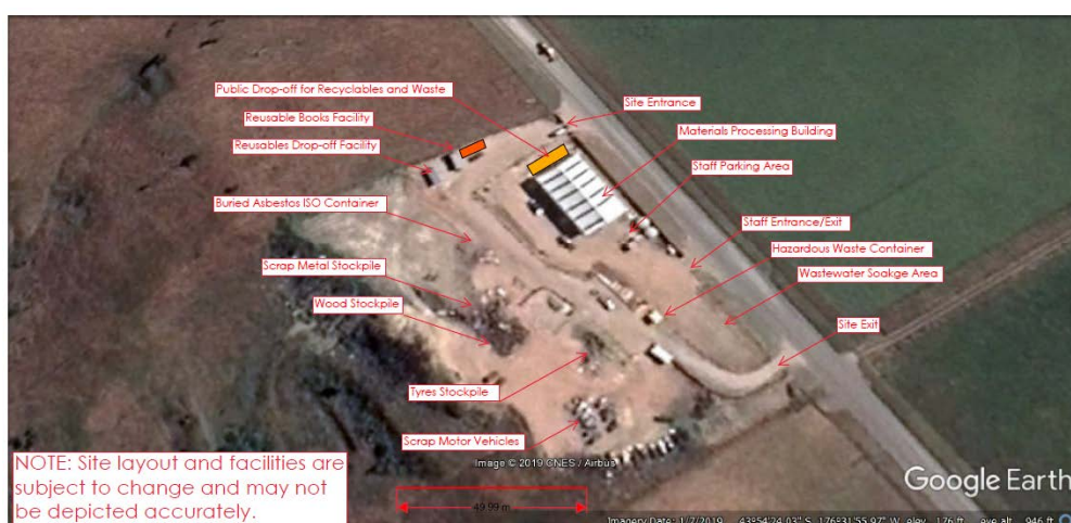
Figure 4 Annotated Aerial Photograph of Te One MRF.
