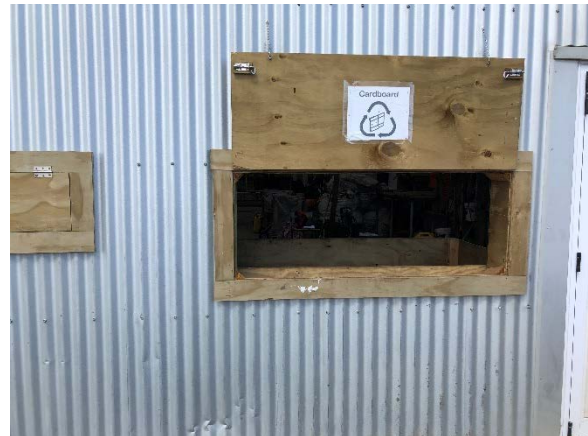
Figure B2-2: Slots installed for placing dry recyclables into fadges.
