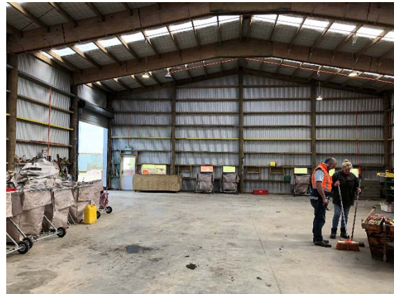
Figure B2-8: Inside the MPB showing recycling “slots” and fadges.
