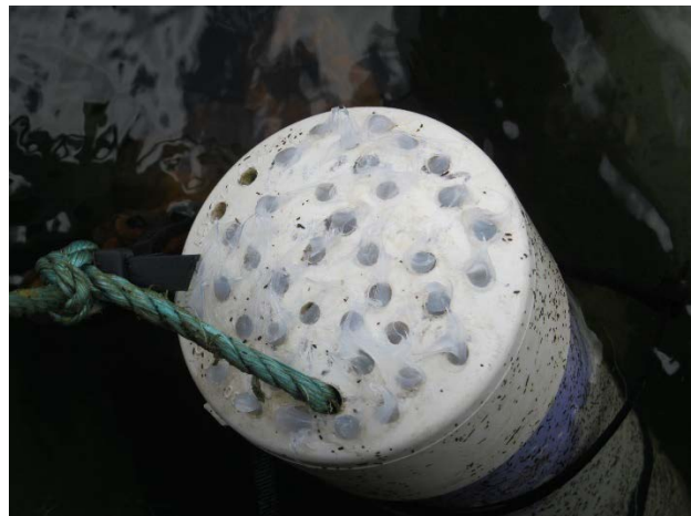
Figure B3-4: Outlet pipe with single hole outlet (other holes are filled with silicon).
