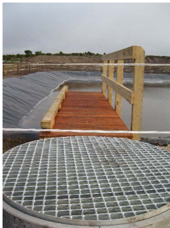
Figure B3-3: Leachate pond outlet structure.
