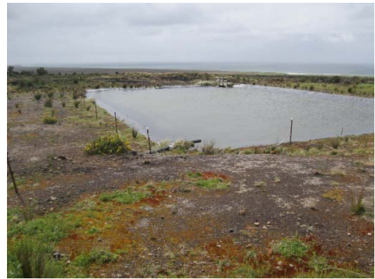
Figure B3-2: Leachate pond.
