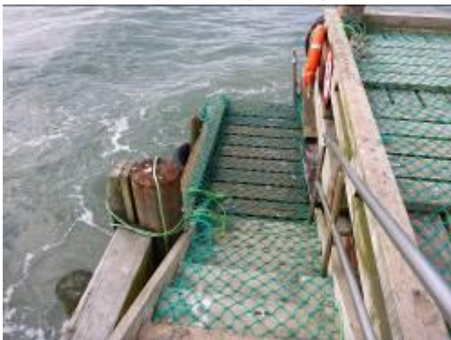
Steps at the end of Owenga wharf.
