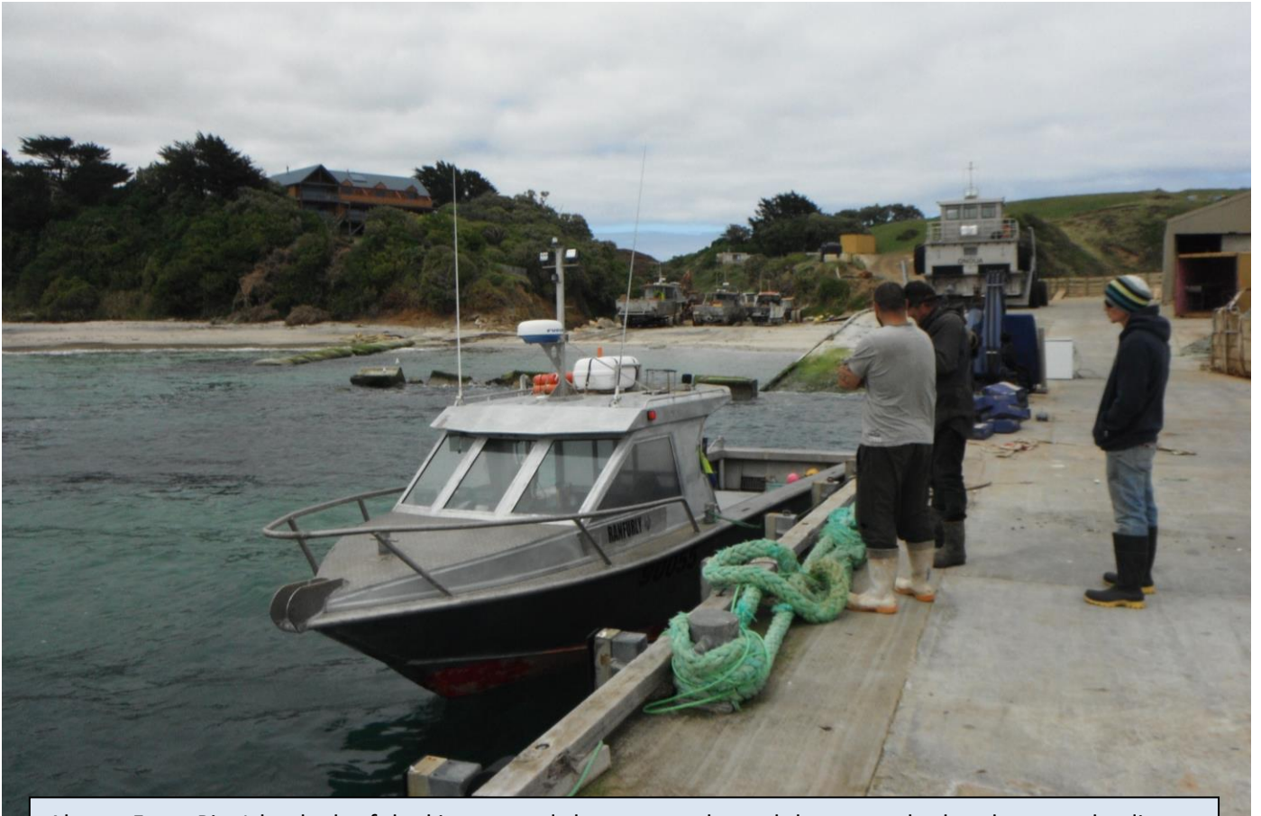
Above: From Pitt Island wharf, looking toward the narrow channel, between the breakwaters, leading to the fishing boat beach.
