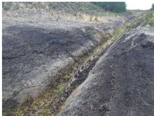
Fig. 54 Pipe from filtration tank to discharge field
