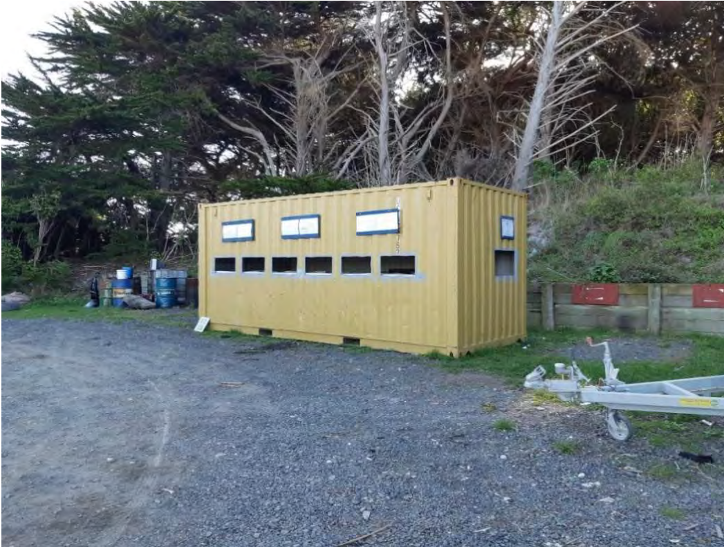
Fig. 56 Kaingaroa Transfer Station
