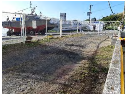
Fig. 84 Concrete pad area for refuelling
