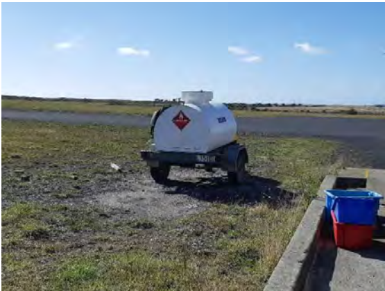
Fig. 30 Mobile Fuel tank (double skinned) stored outside bunded area
