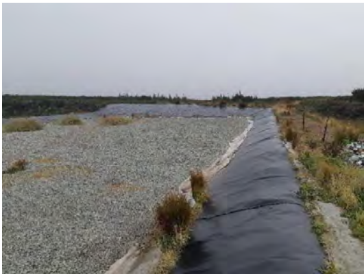
Fig. 51 Sorted waste storage site
