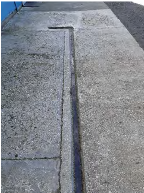
Fig. 25 Factory and stormwater channel
