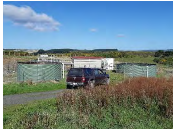
Fig 103. Waste water treatment plant
