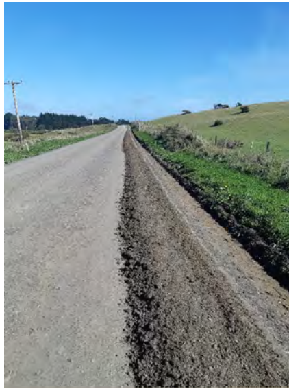
Fig. 64 Gravel road grading in progress.
