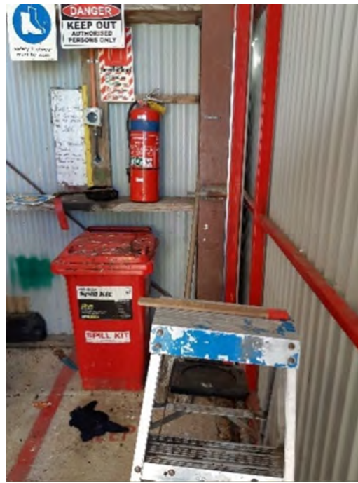
Fig. 33 Spill kit present in adjacent building
