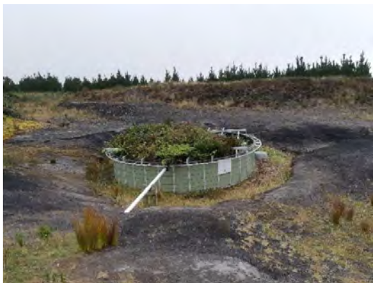
Fig. 53 Filtration tank
