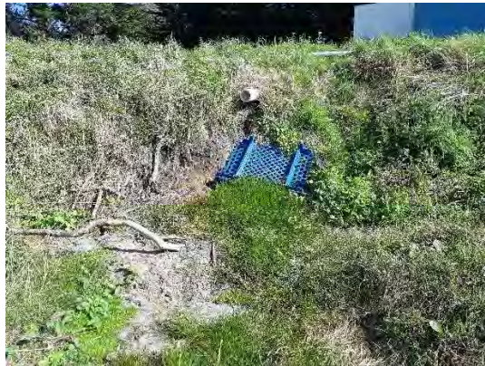
Fig. 26 Stormwater discharge pipe into stream bank
