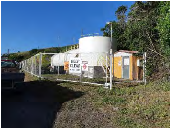
Fig. 80, 81 Bulk fuel storage 400,000 litres diesel in bunded area
