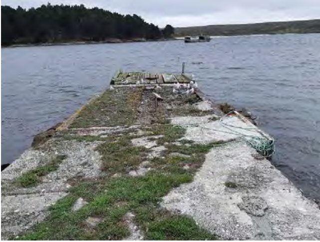
Remaining part of Port Hutt wharf
