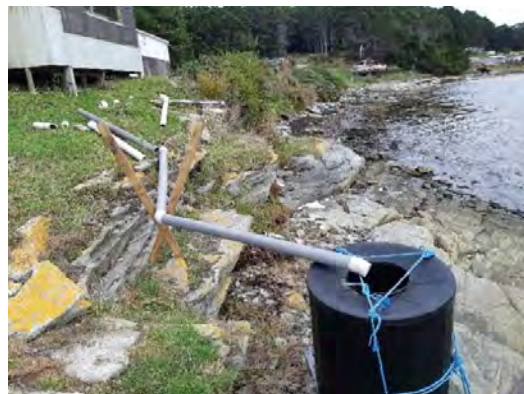
Fig. 11 Makeshift tank for chemical washdown discharge from factory
