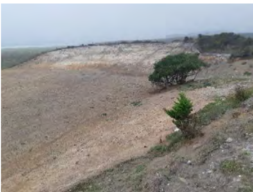
Fig. 45 Recently closed landfill (overview from top)
