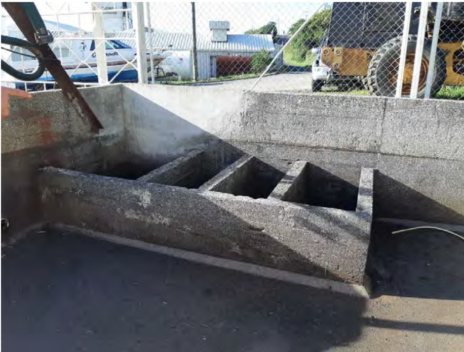
Fig. 85 Bunded area near refuelling pad
