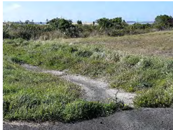
Fig. 34 & 35 Open stormwater drainage channels off runway into ground and lagoon
