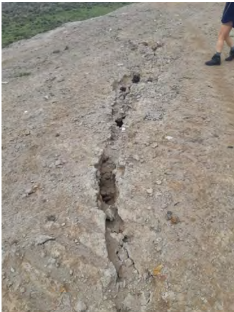
Fig. 44 Cap failure/erosion
