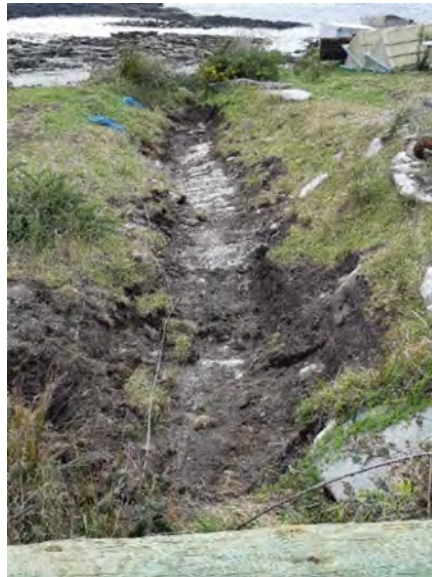
Fig. 16 Recent remediation of diesel spill
