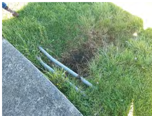
Fig. 70 Stormwater discharge point to creek behind concrete pad.
