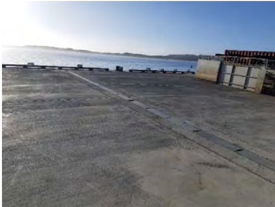
Fig. 76 & 77 Stormwater strip drains leading to shut off valve (then sea)
