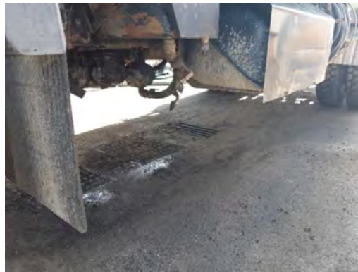
Fig 68. Tanker fuel leak on bunded area
