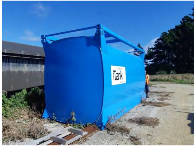
Fig. 3 New double skinned fuel containment awaiting installation
