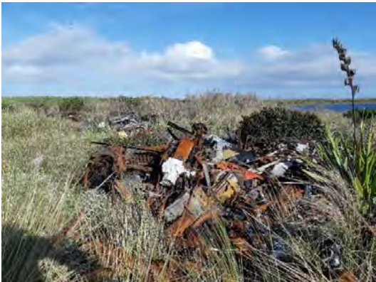
Fig. 49 Exposed refuse through landfill cap
