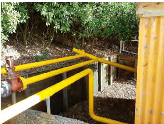
Fig. 81 and 82 Overground fuel line to bulk storage
