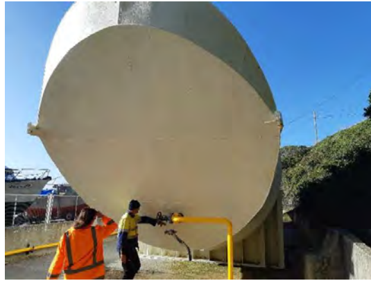
Fig. 80, 81 Bulk fuel storage 400,000 litres diesel in bunded area
