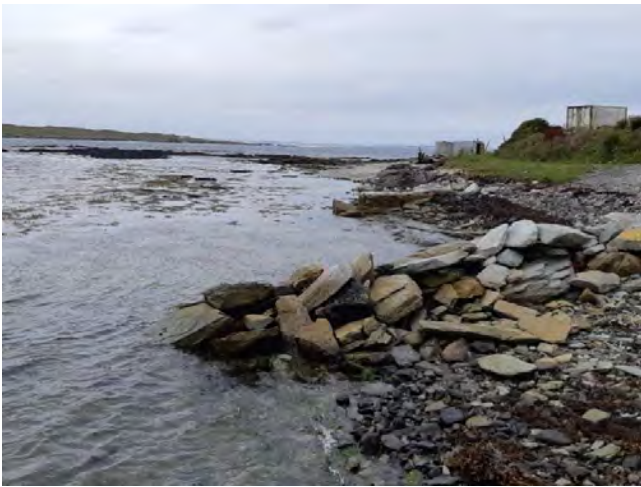
Fig. 91 Port Hutt vessel slipways
