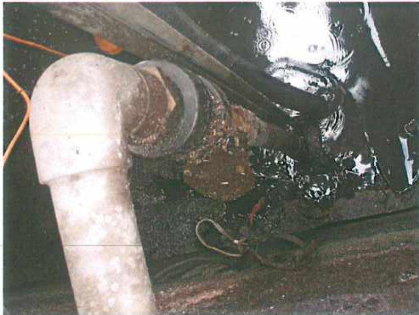
Corroded check valve at main pump station
