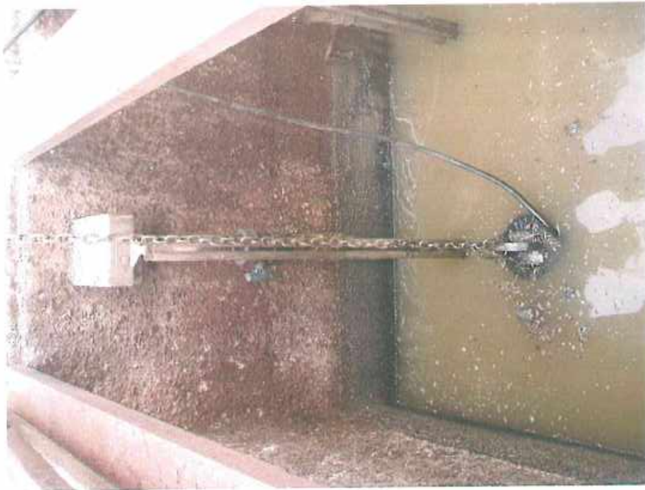
Faulty pump in wet well
