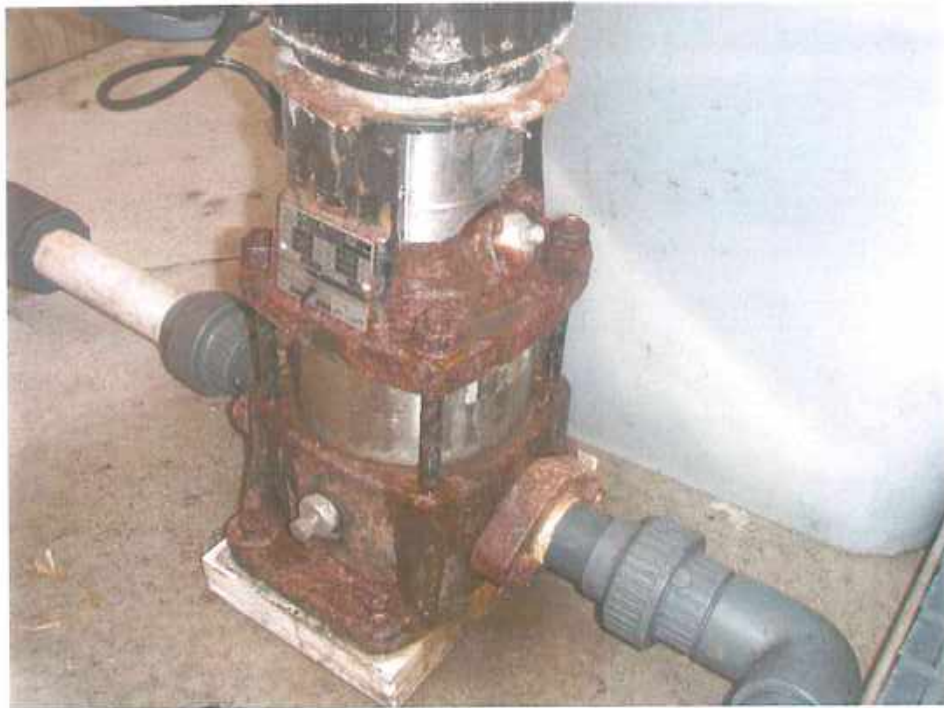
Leaking pump at Kaingaroa
